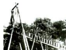
Fig. 3. Pulse voltage generator for output voltage 3.5 MV for lightning resistance tests of aerial power lines Donbassenergo, 1934
